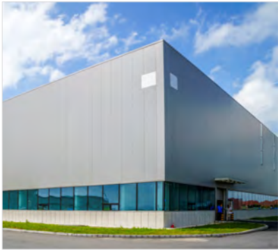
ACP UNIT-3 Hindupur, Andhra Pradesh
